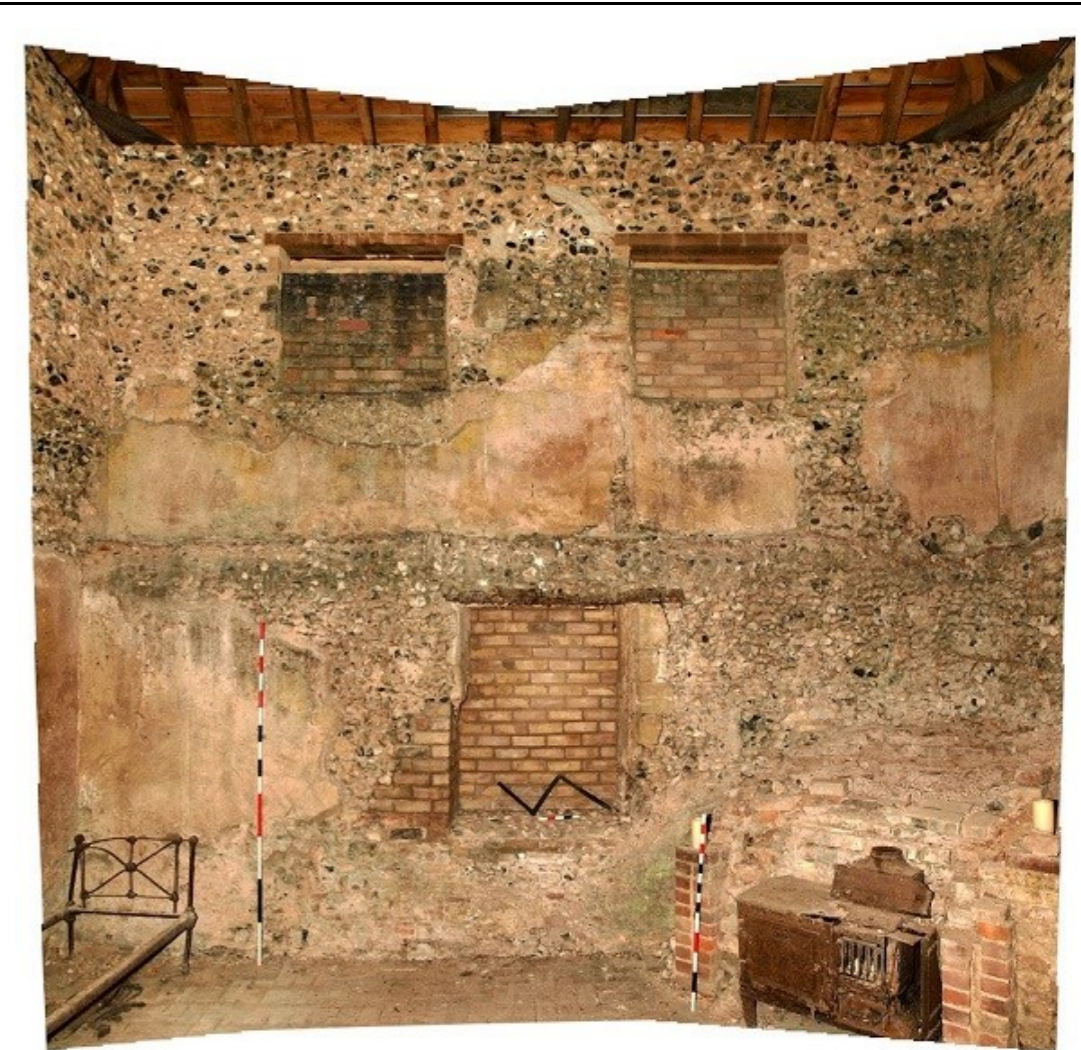
Internal south face of Mildenhall Warren Lodge. Photo: James Cross (May 2017)
