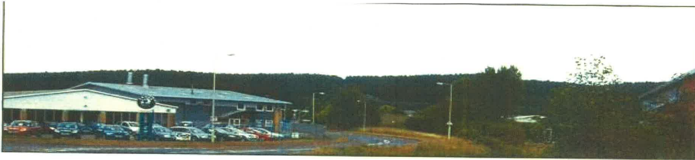
Photograph 3: View from Winner Garage on Valley Road looking east
